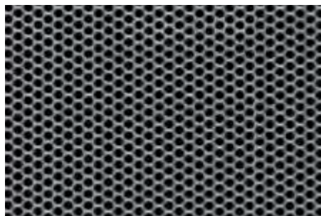
(PARKING GARAGE WALLS ONLY) PERFORATED METAL INFILL PANELS, PAINTED TO MATCH COPING
